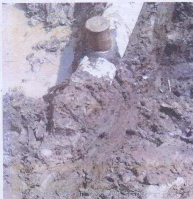
Fig C: Incident facility during repairs
