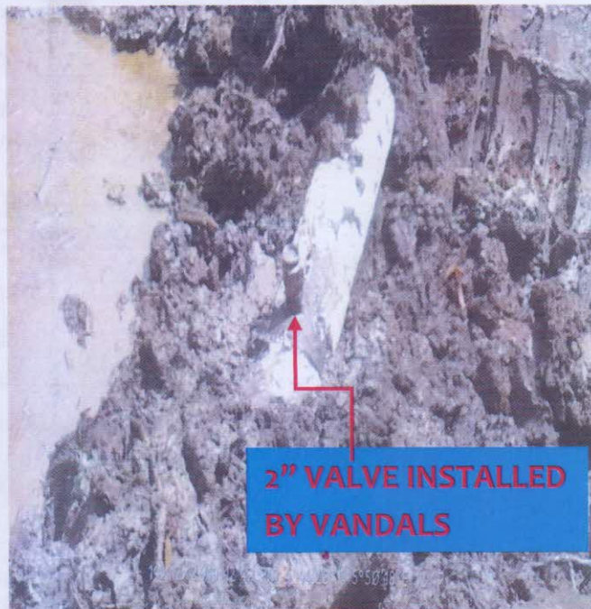
Fig B: Incident Facility after excavation
